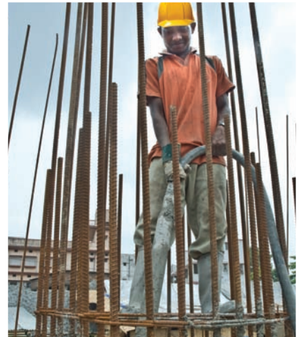
Use of vibrator for compaction
