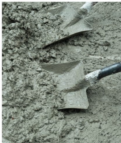
Concrete mixing on impervious platform
